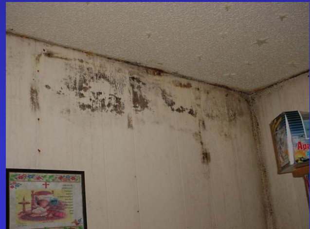
Mold due to leaky roof
